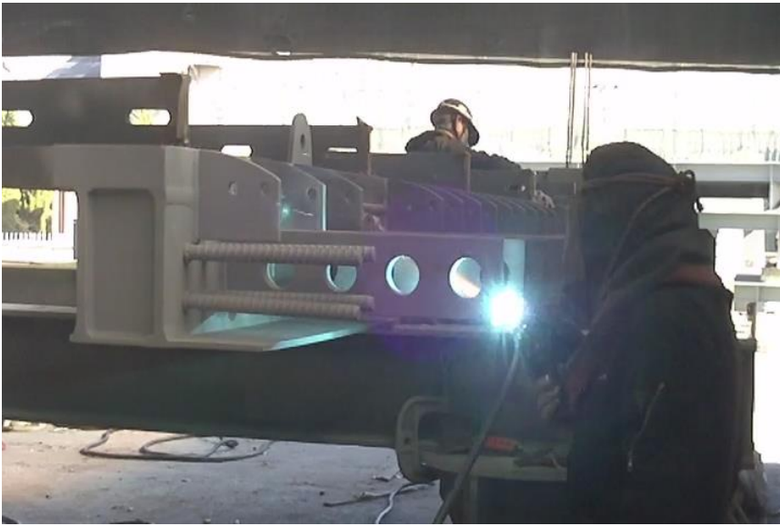
(橋梁連結部溶射)
